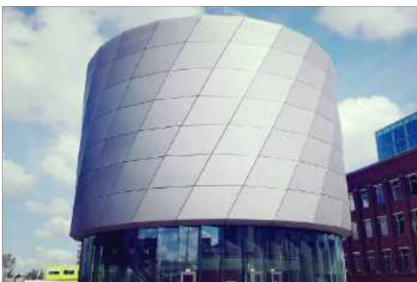
Gevelbekleding This Is Holland paviljoen
