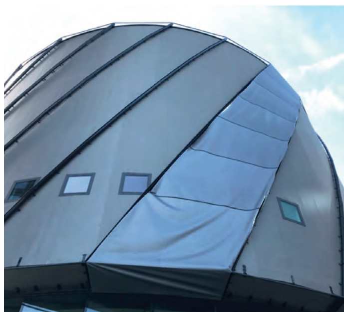
De gevelbekleding is in diagonale stroken gespannen. (Foto: Buitink Technology)
