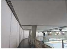
Ceiling and walls Vaujany ice rink (FR)
