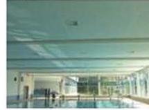
Tensioned ceiling Aqua centre (CH)
