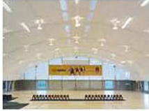
Tensioned ceiling Sports hall (NZ)
