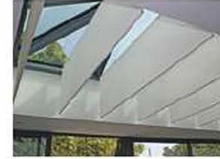
Ceiling and baffles Restaurant (FR)
